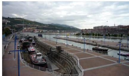
Muelle Churruga Quays
